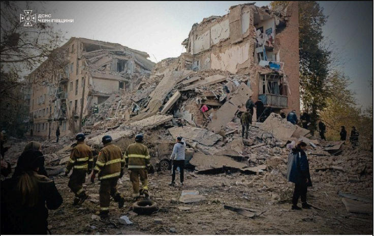
Rescuers at the collapsed section
