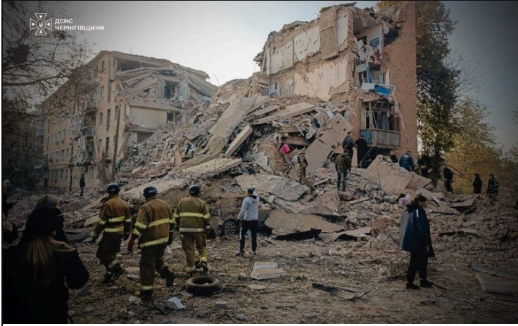
The collapsed entrance section
