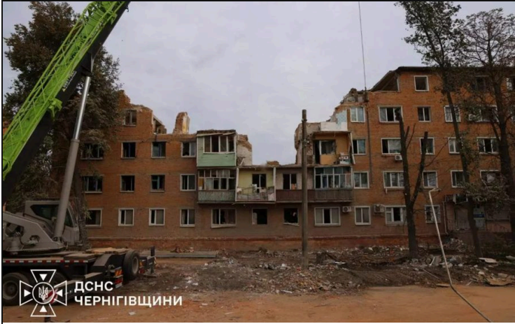
Pryluky: the residential block after the strike; search and rescue continued until 8 October
