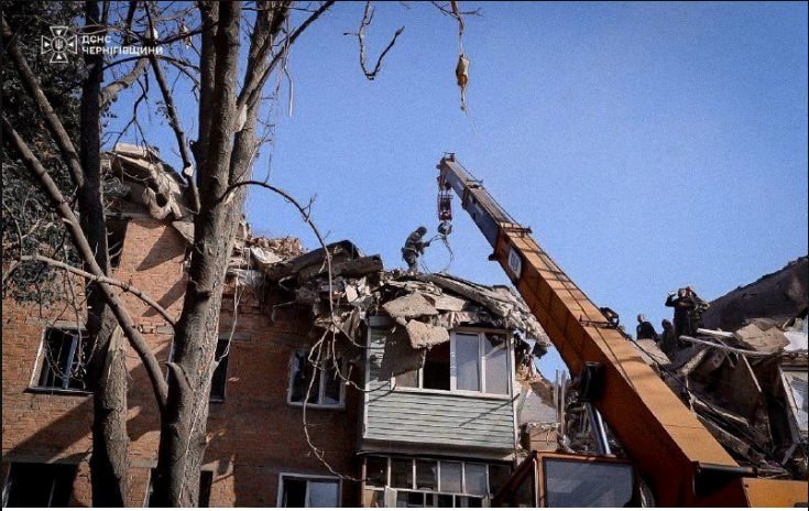
A crane lifts slabs during the search
