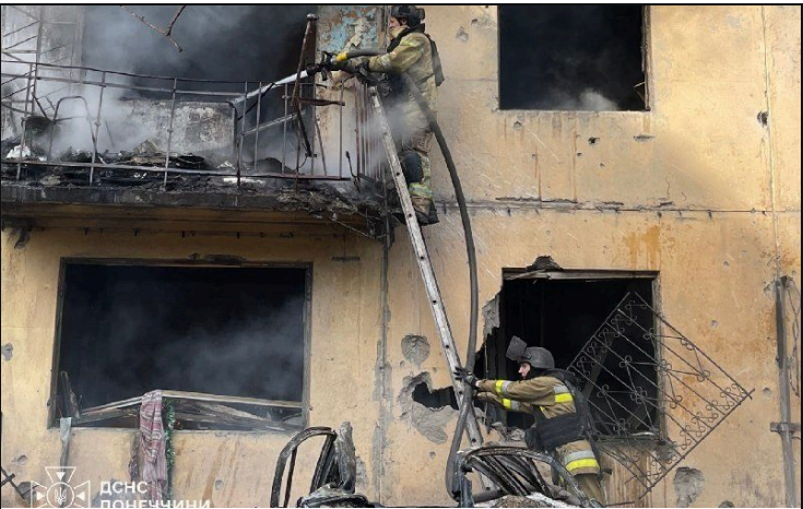
Kramatorsk, 20 Oct: rescuers on a burnt-out balcony of the same block State Emergency Service of Ukraine (DSNS) · 2026-10-20 · CC BY 4.0 https://t.me/dsns_telegram/78241
