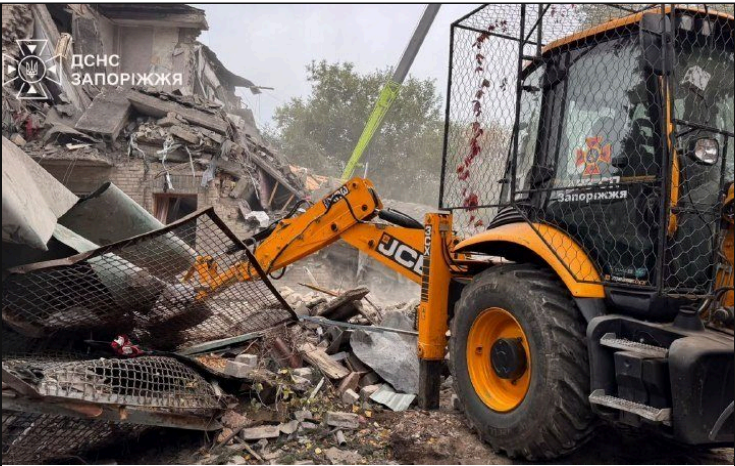
An excavator clears the collapsed section
