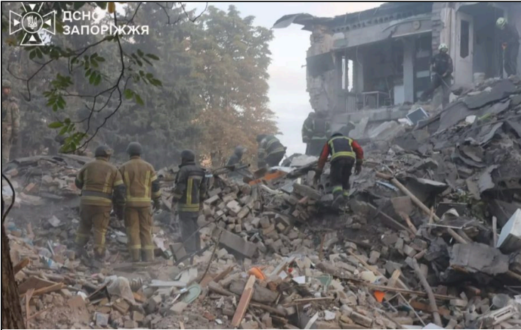
Zaporizhzhia: rescuers on the collapsed entrance section, 11 October
