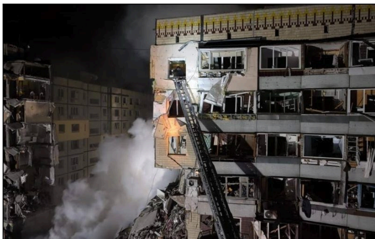
Rescuers at the collapsed entrance at night
