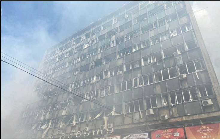
The office block opposite, its windows blown out State Emergency Service of Ukraine · 2022-07-14 · CC BY 4.0 https://commons.wikimedia.org/wiki/File:Vinnytsia_after_Russian_shelling,_2022-07-14_(03).jpg
