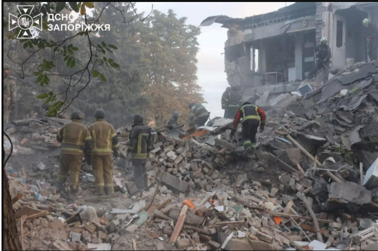
Zaporizhzhia, 11 Oct: rescuers on the collapsed entrance section. Photo: State Emergency Service, Zaporizhzhia region · CC BY 4.0 · zp.dsns.gov.ua
