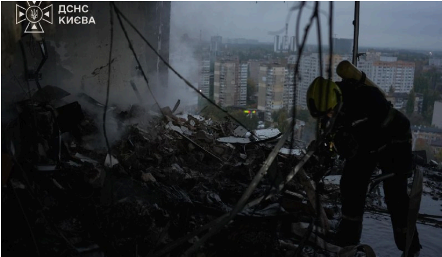
Rescuers in the burnt-out apartment on the 20th floor, 21 Oct. Photo: State Emergency Service of Ukraine (DSNS) · 2026-10-21 · CC BY 4.0
