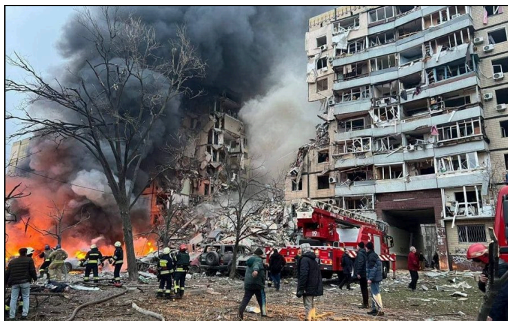
The nine-storey block on Naberezhna Peremohy Street burning after the strike, 14 January 2023
