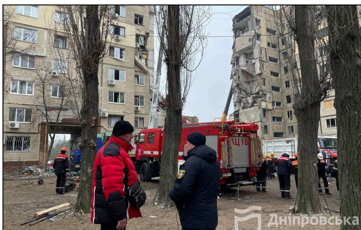
Residents and rescuers outside the building
