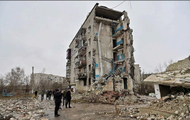
2 Pershotravneva St: the collapsed section of the building
