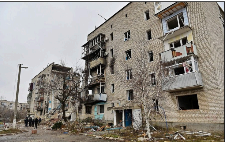
The apartment block at 2 Pershotravneva St, struck on 9 Mar 2022
