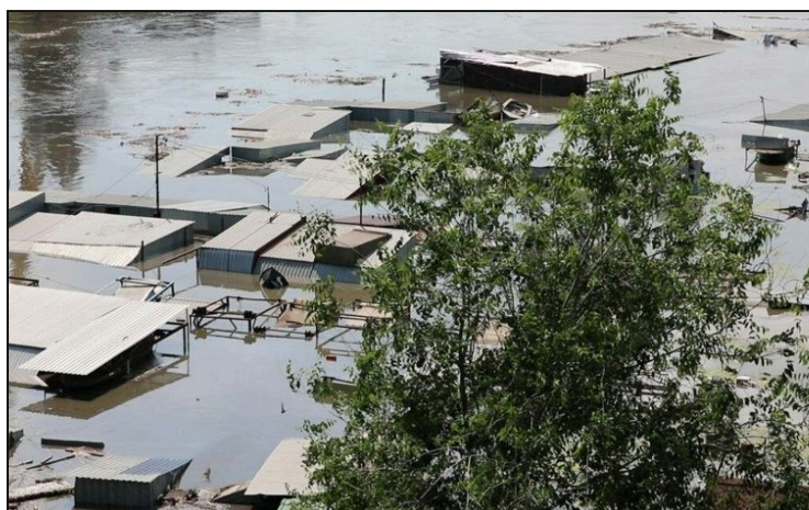
Settlements on the left bank under water after the dam was destroyed, June 2023
