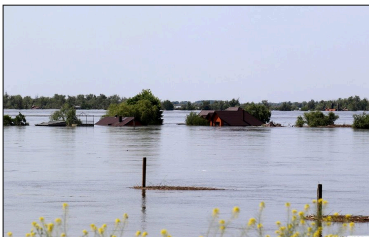
Kherson the day after the dam was destroyed, 7 June 2023
