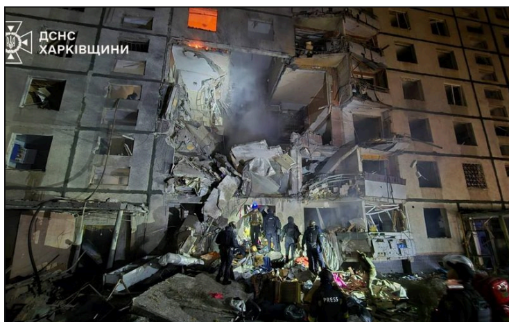
The collapsed stairwell of the nine-storey block in Saltivskiy district, Kharkiv, during the night rescue, 31 October 2024
