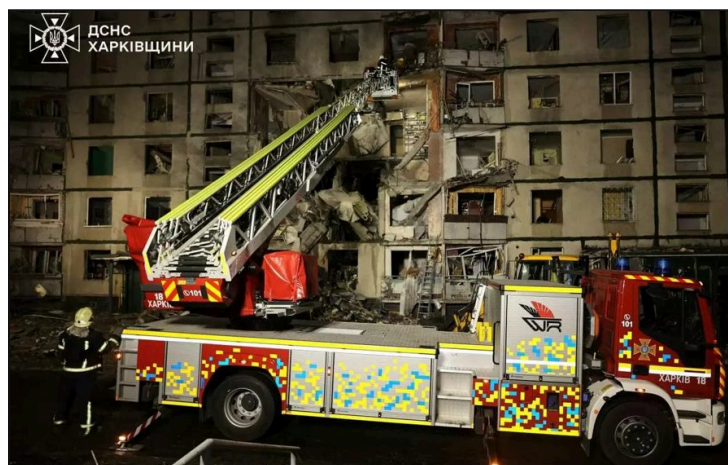
A State Emergency Service ladder truck at the damaged block, night of 30–31 October 2024
