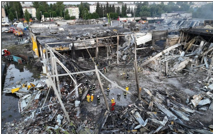
The ruins of the shopping centre the next day, 28 June 2022
