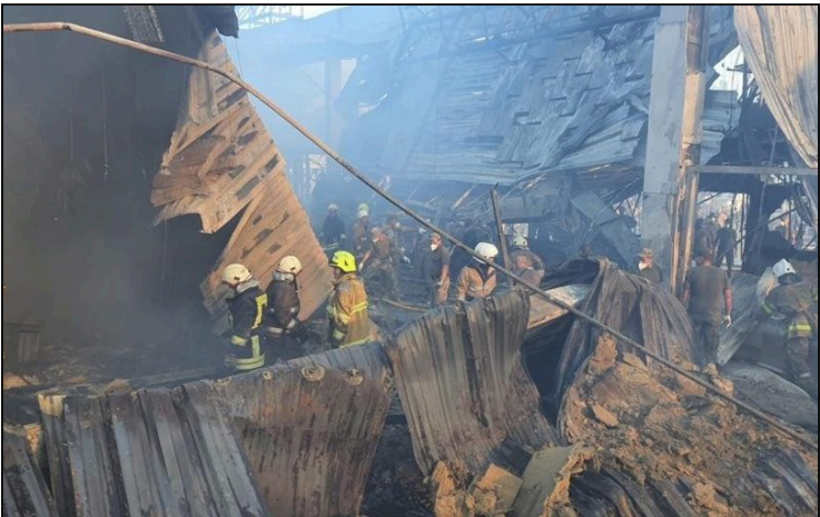
Rescuers in the collapsed structure
