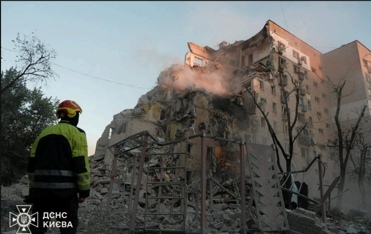
The collapsed section of the apartment block in Darnytskyi district
