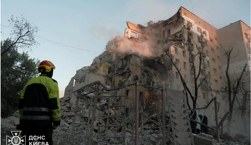
The collapsed section of the apartment block in Darnytskyi district. Photo: State Emergency Service of Ukraine · CC BY 4.0 · via Wikimedia Commons
