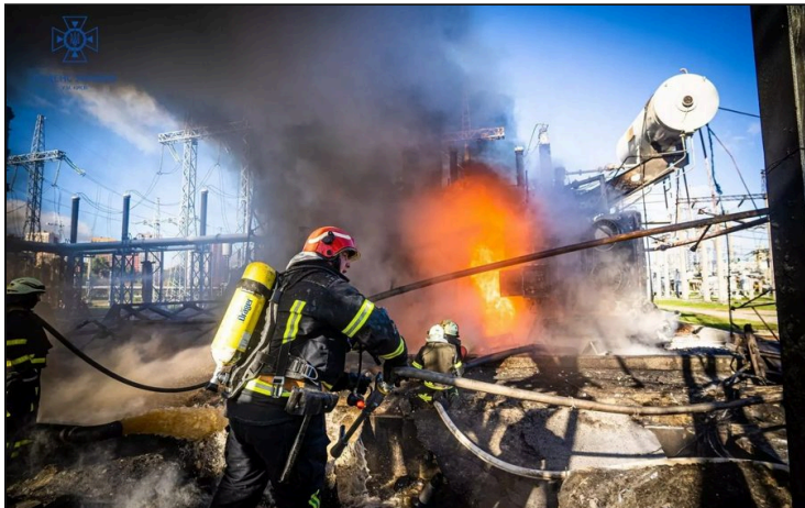
A combined heat and power plant in Kyiv on fire after Russian missile strikes, 10 Oct 2022 — three weeks before the strike that cut water
