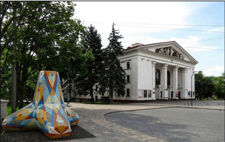
The theatre and Theatre Square before 2022
