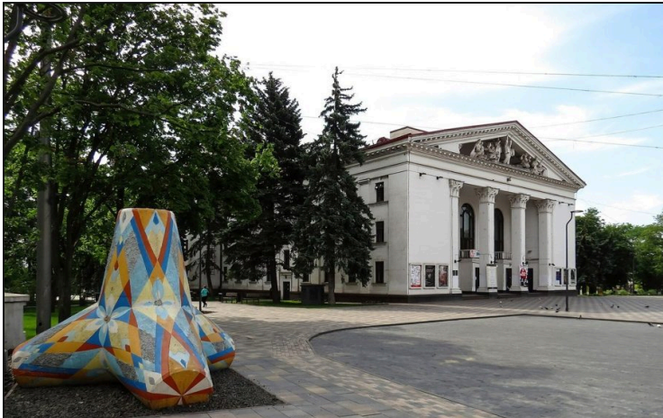
The theatre and Theatre Square before 2022
