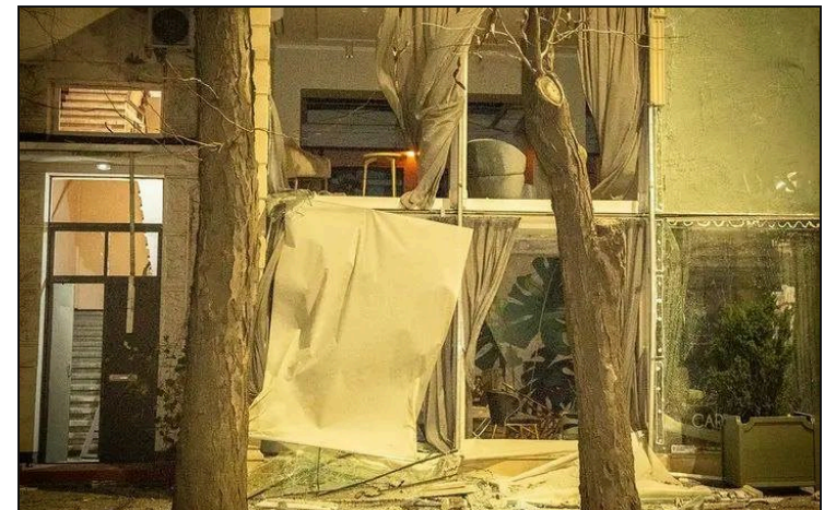
A shopfront blown out by the blast wave in the historic centre, 6 November 2023
