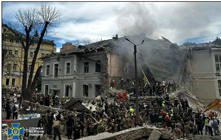
The destroyed toxicology building of Okhmatdyt
