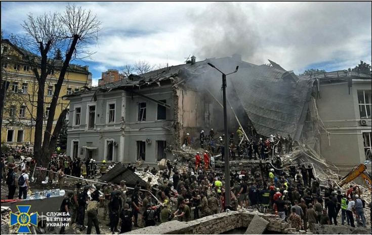
The destroyed toxicology building of Okhmatdyt
