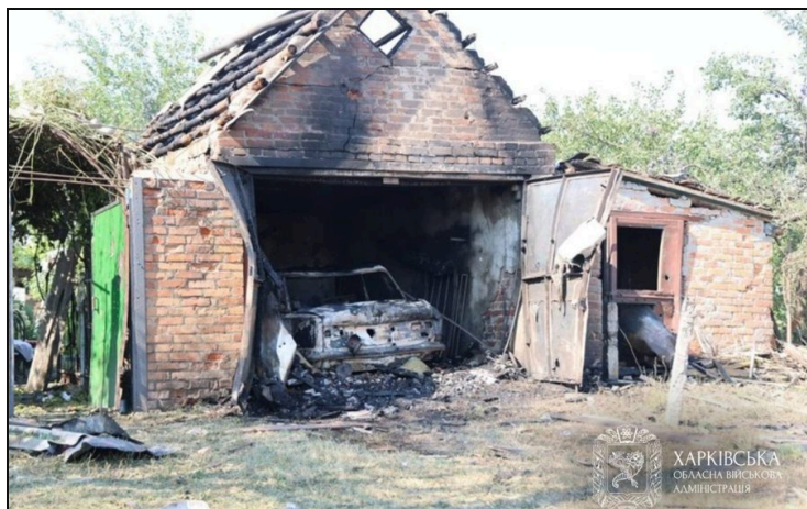
The centre of Pechenihy after the missile strike of 18 August 2026 — regional administration release, frame 4 of 6
