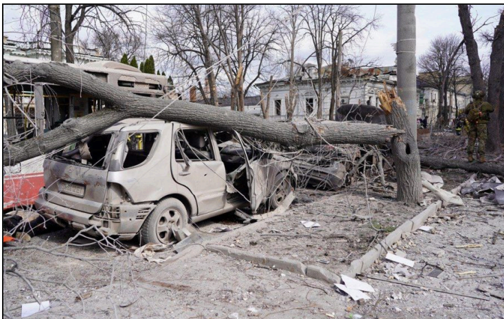
Destruction in central Sumy on the morning of Palm Sunday
