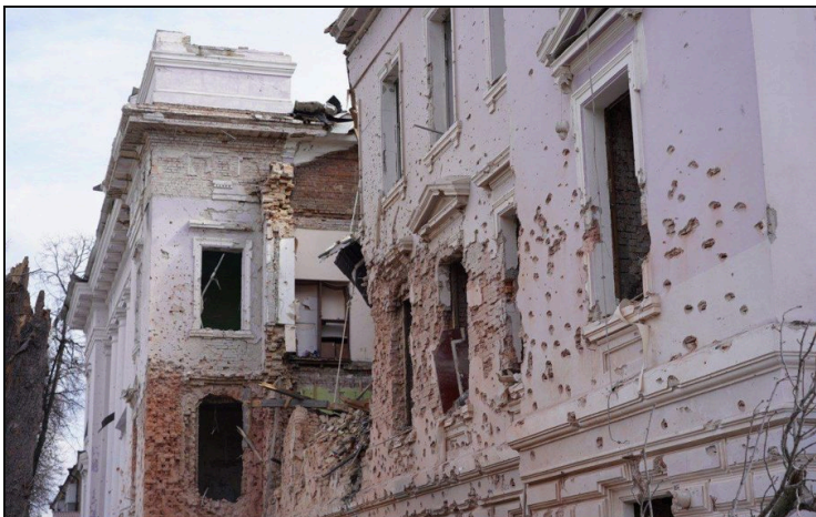
A building of Sumy State University, Petropavlivska Street 57, after the strike
