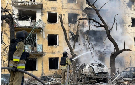
Kramatorsk: the site after the strike · State Emergency Service of Ukraine (DSNS) · 2026-10-20 · CC BY 4.0
