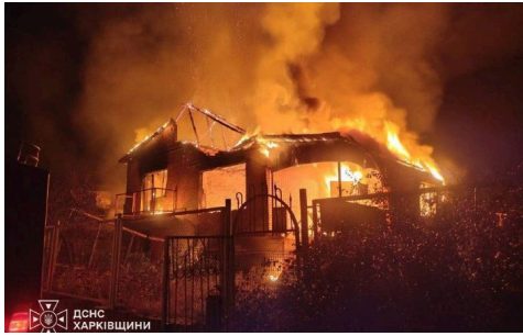
Izioum: the site after the strike · State Emergency Service of Ukraine (DSNS) · 2026-10-20 · CC BY 4.0
